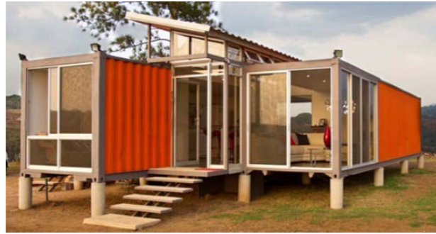
Figure 3. Cargo container home using precast pile foundation 5 .
