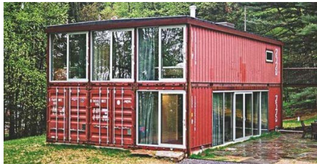
Figure 5. Cargo container home secured with original corner fittings 8 .
