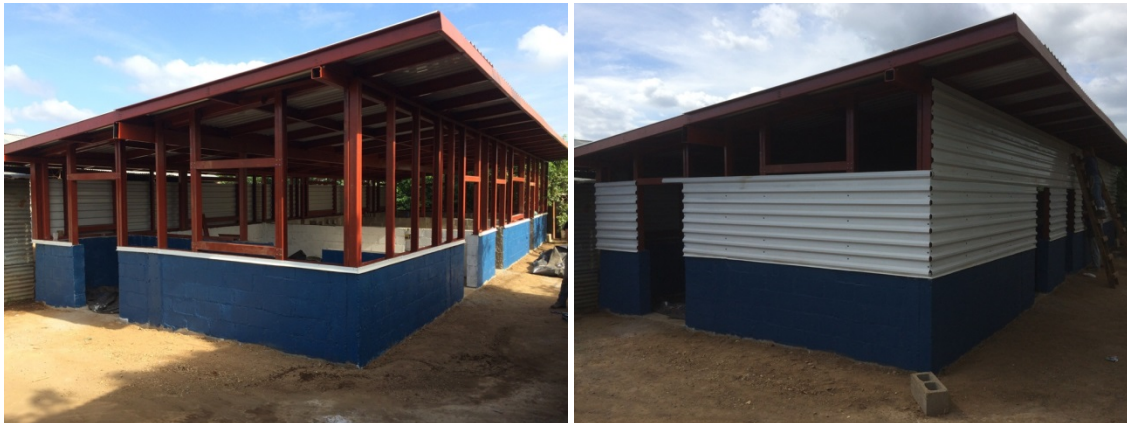
Figure 16 The structural system (left) and cladding (right)
