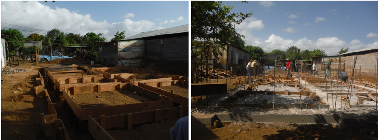
Figure 18 Foundation construction before (left) and after (right) placing concrete
