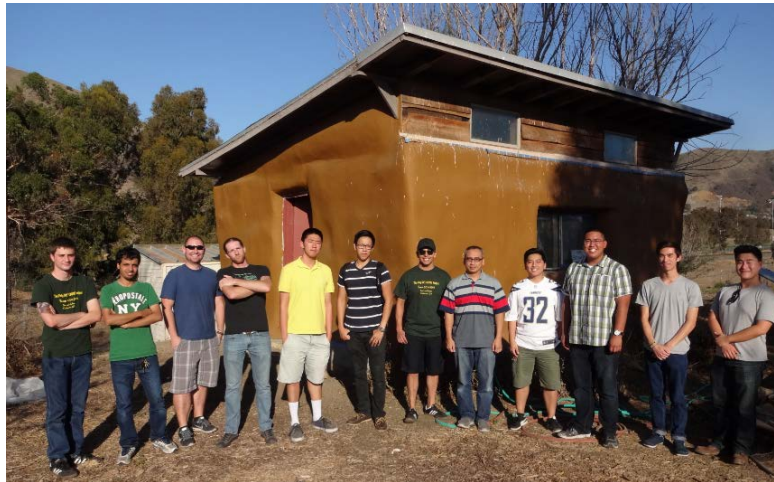
Figure 2. This figure shows the DC House prototype at Cal Poly State University
