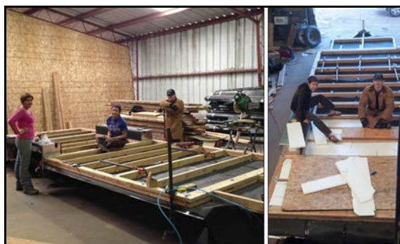
Figure 4. Tiny house under construction.
