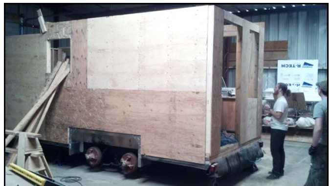
Figure 9. Vagabond House, walls going up!
