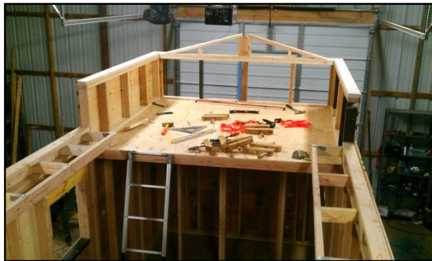
Figure 13. Vagabond House loft & framing.
