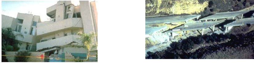
Figure 1. Structural failures of building and bridge in the 1994 Northridge earthquake.
