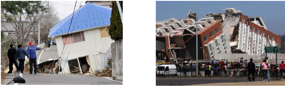
Figure 2. Structural damages in 2011 Japan earthquake.
